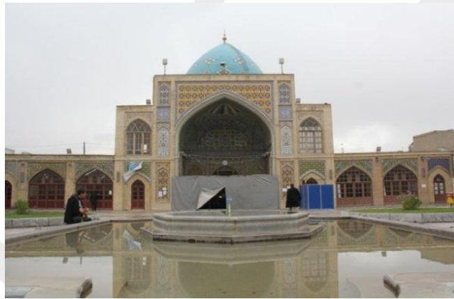
Figure 1. A view of Jameh Mosque of Zanjan (Photo taken by author)
