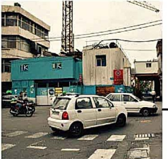
Line 6 of subway which is in construction
