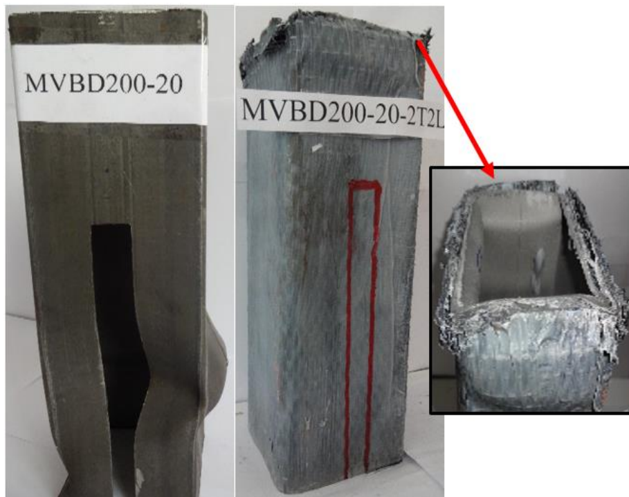
Fig. 10. Failure modes of the specimens with middle-bottom deficiency: non-strengthened and strengthened
